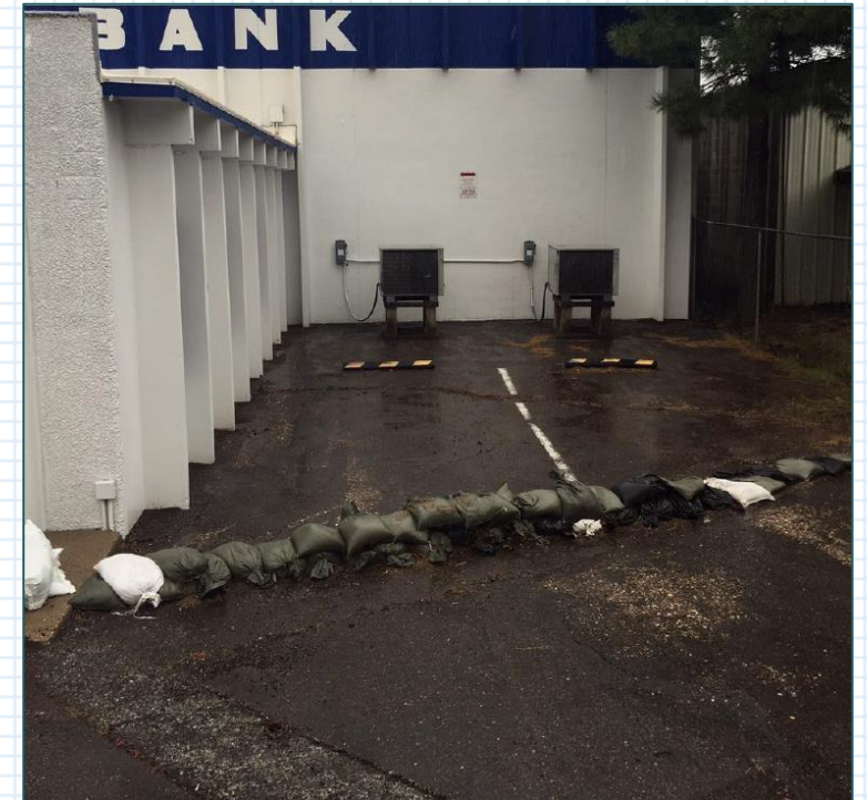
Figure 12: Further Flooding Prevention (Sandbags)
