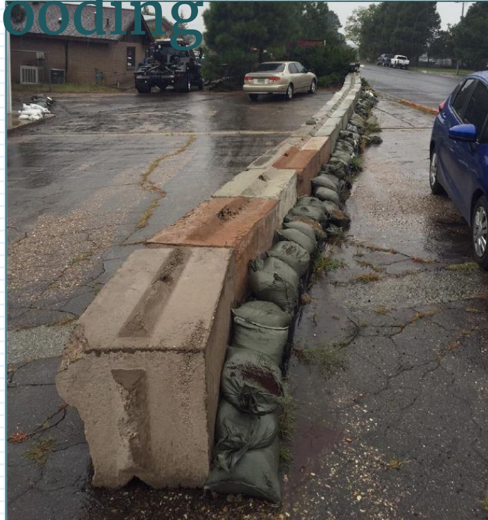
Figure 11: Front Concrete Barricades
